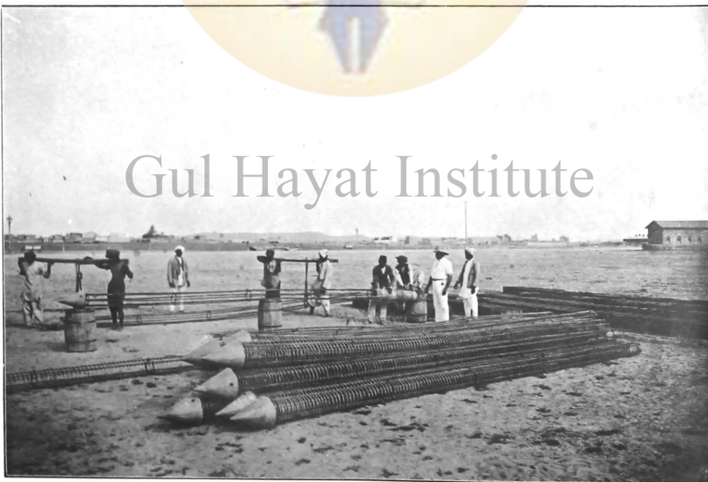
12—New Customs House, Karachi—Cores for piles.
