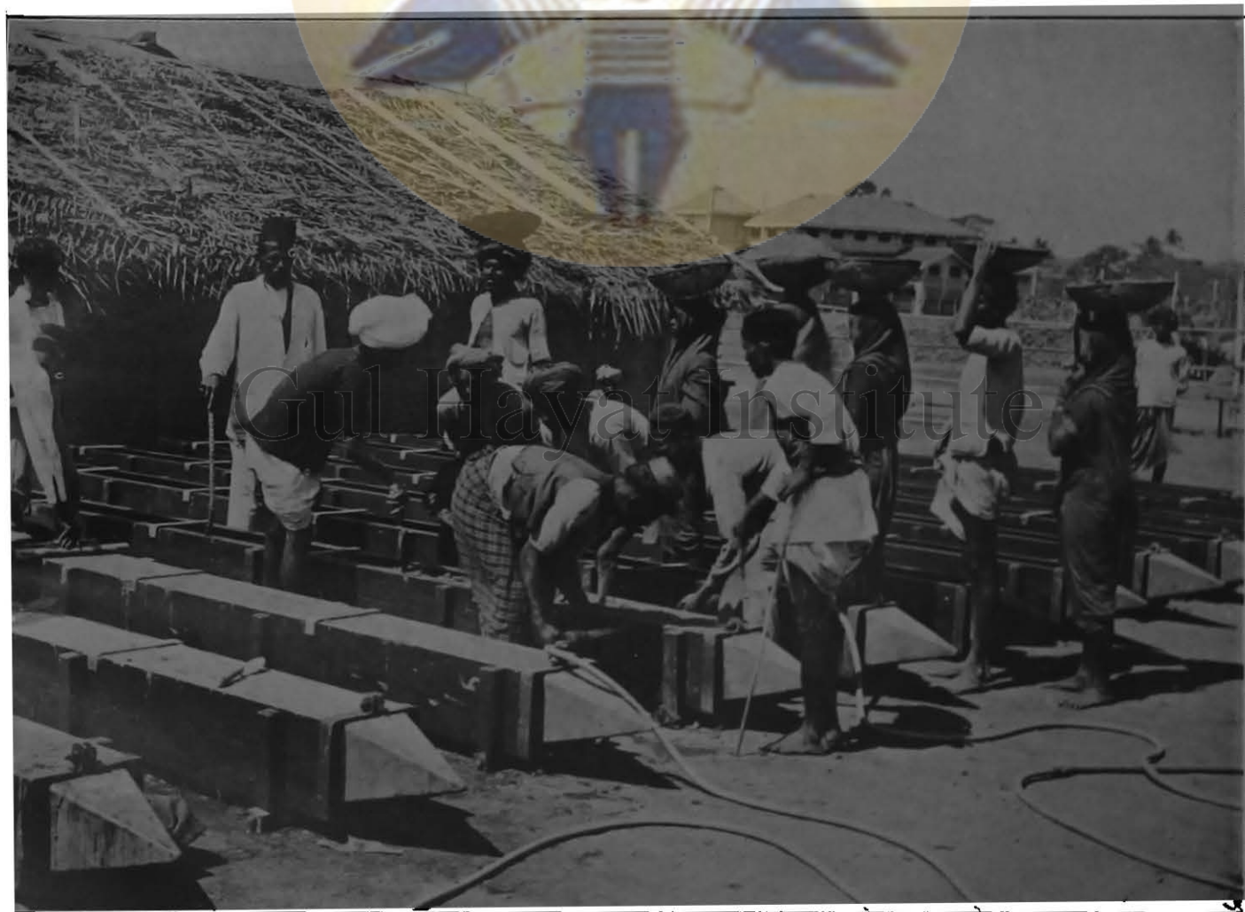
6—Kennedy Sea Face, Bombay—Filling reinforced cement concrete piles, showing method of vibrating the moulds with pneumatic hammers. 21st March 1915. Work commenced—20th February 1915. Number of piles completed upto 21st March 1915—77.
