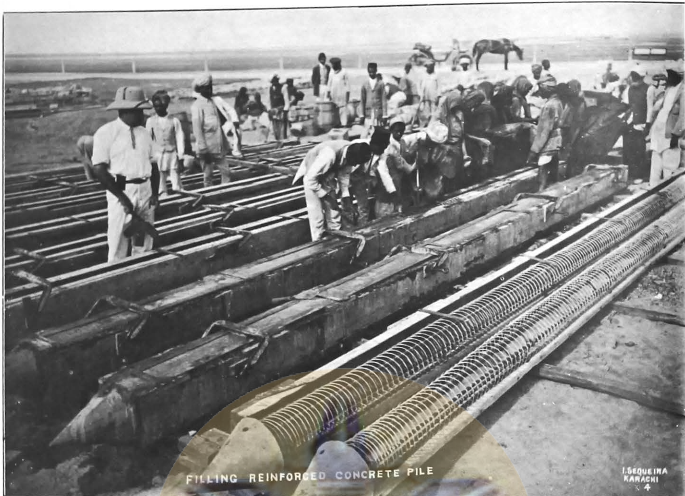
11—New Customs House, Karachi—Filling reinforced concrete piles.
