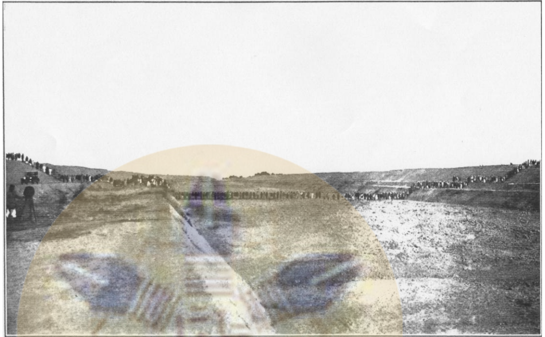
'View of North Western Perennial Canal – Mile 8, near Bagarji. Designed discharge 5,152 cusecs. Bed width 165 feet. Depth of water 10.2 feet', N.a., The Opening of The Lloyd Barrage and Canals , p.28.
